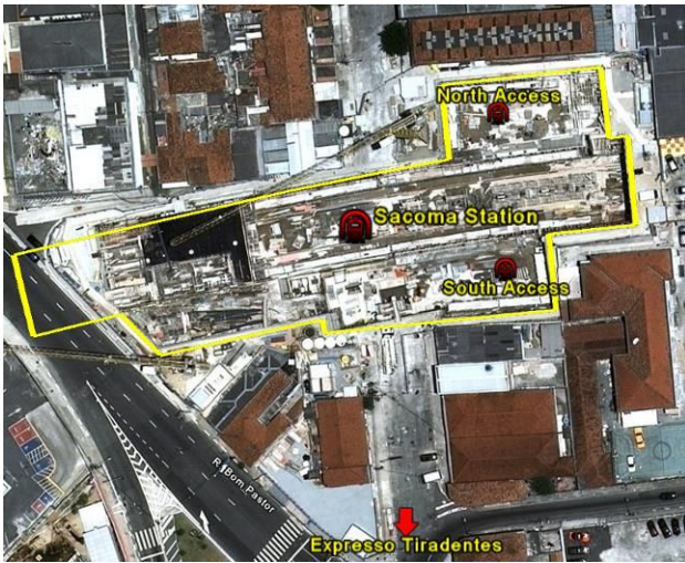
Figure 10. Aerial view of station's work site.
