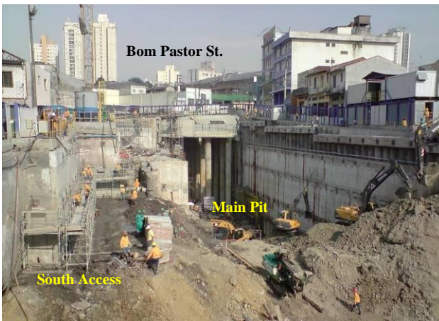
Figure 11. South access pit on the left and main excavation of station.
