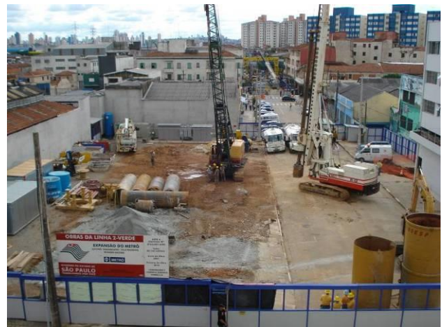
Figure 5. Station's vicinity before excavation.
