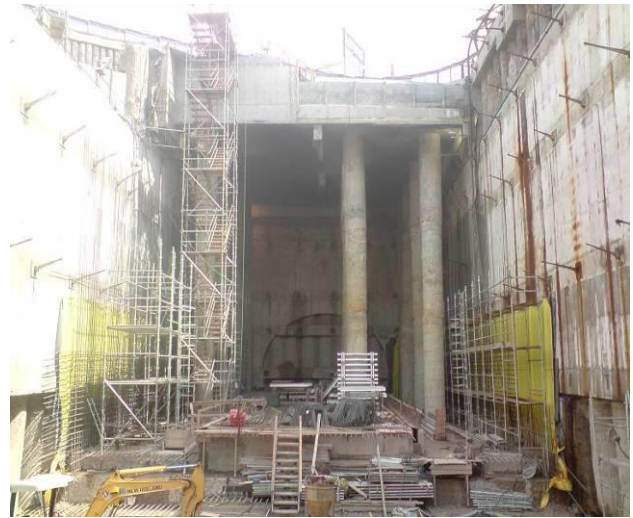
Figure 12. Top-down excavation below Bom Pastor Street.
