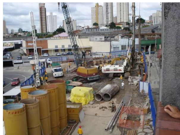
Figure 6. A different angle of station's vicinity before excavation.
